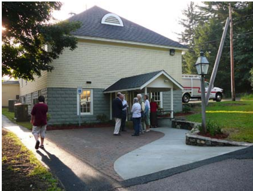
New Accessible Parking Spot and Walk
