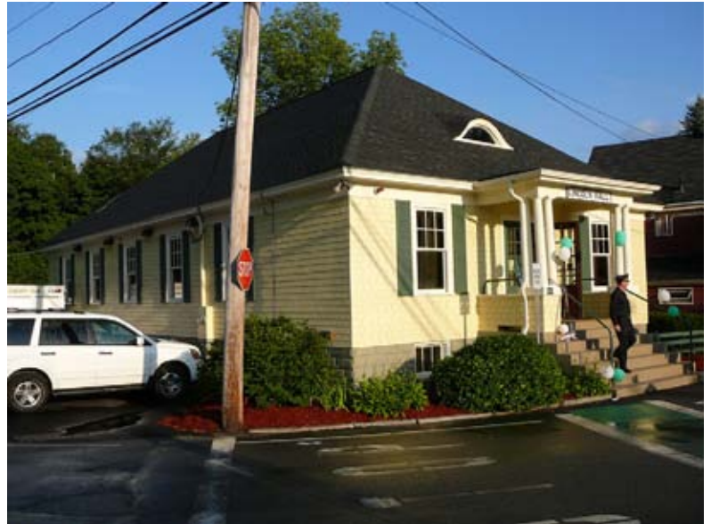
Photograph of Complete Construction
